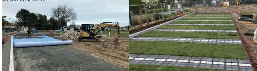
Installation of the active oil-biodegrading aquatextile TenCate GeoClean® under the parking spaces
