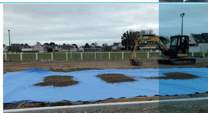
The active oil-biodegrading aguatextile, TenCate GeoClean®, is laid both at the bottom of the swale under a 40cm thick coarse gravel layer and under the parking spaces with permeable pavement.
