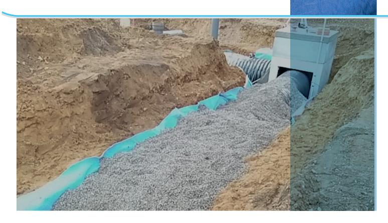
□ Oil separator: requires a single injection point and treatment, before being discharged into the infiltration structure. The configuration of the project was unsuitable for this intervention and it was impossible to provide a sectioning and containment valve.
